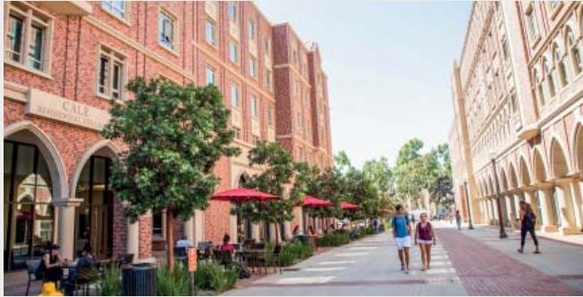
CALE AND IRANI RESIDENTIAL COLLEGE (UVS) (CIC) 929 West Jefferson Boulevard, Los Angeles 90089
